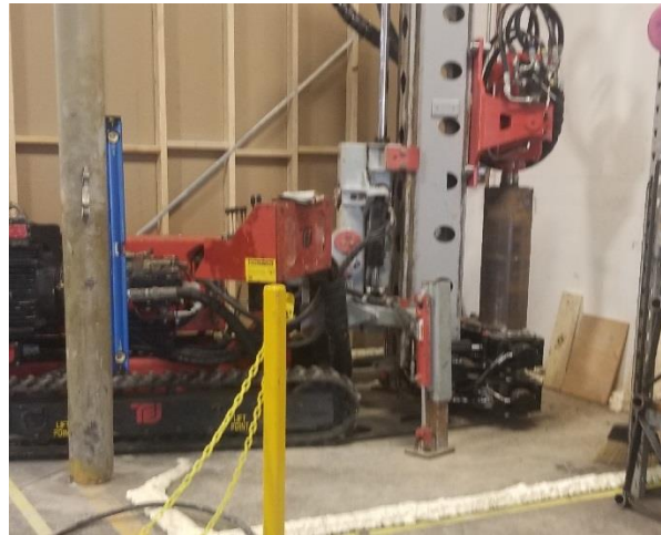
Photo#2 Electric Powered Track Drill
