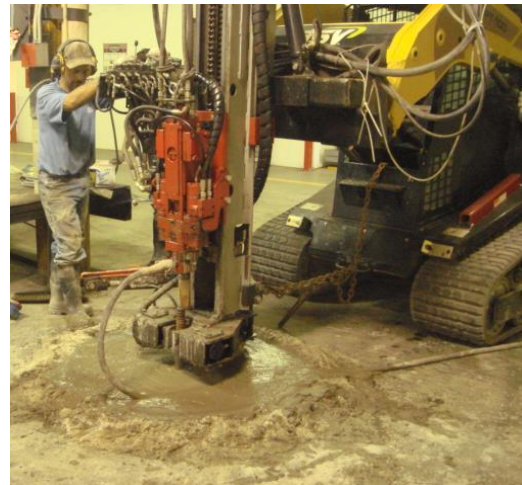
PHOTO#6 Installation inside working area
