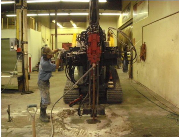
Photo#1 HCM Hydraulic Percussion Drill
