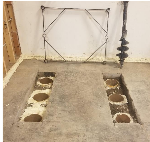
PHOTO#16 Quick tubs installed
