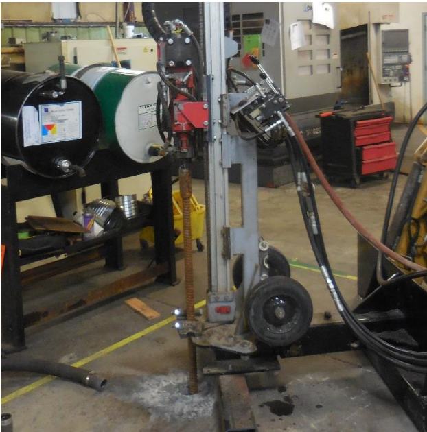
PHOTO#13 Cleaned hole flushing with air
