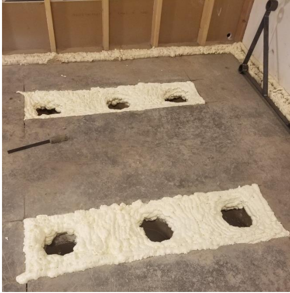
PHOTO#17 Foam cover for piles
