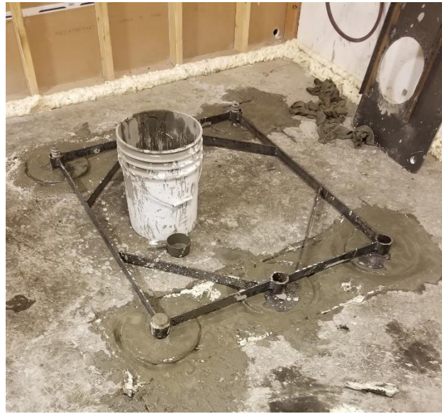
PHOTO#18 Fixture used for pile alignment.
