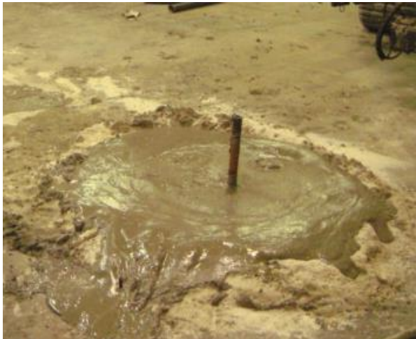
PHOTO#5 Finish Grout around 40mm pile
