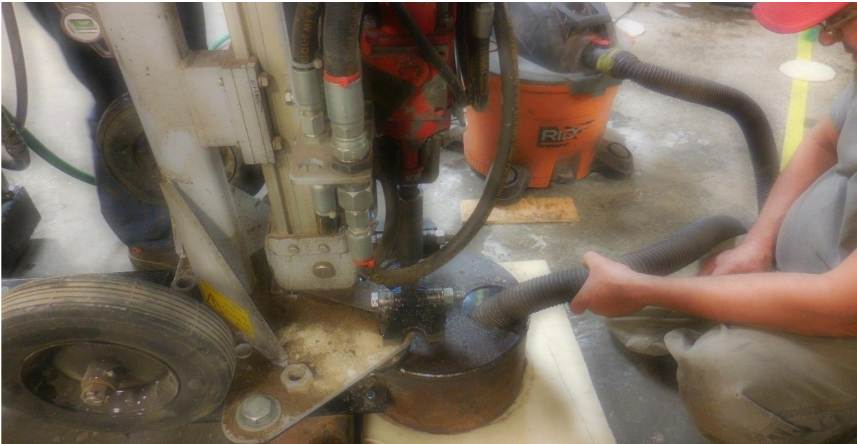
PHOTO#11 Special collector used to collect cuttings while coring the concrete.
