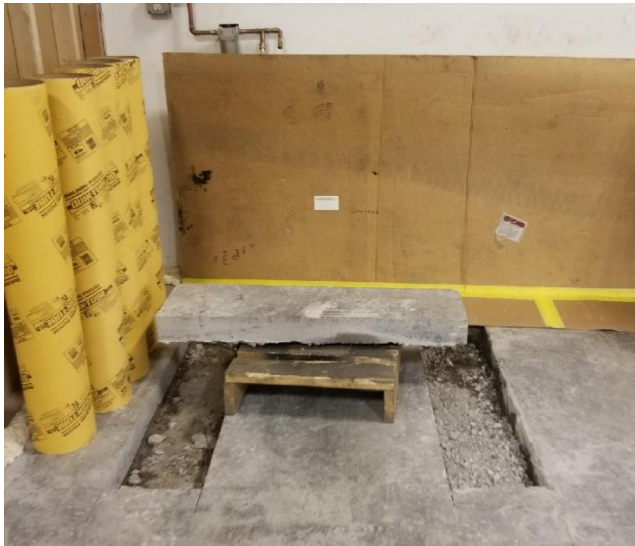
PHOTO#15 Cut out of concrete pad
